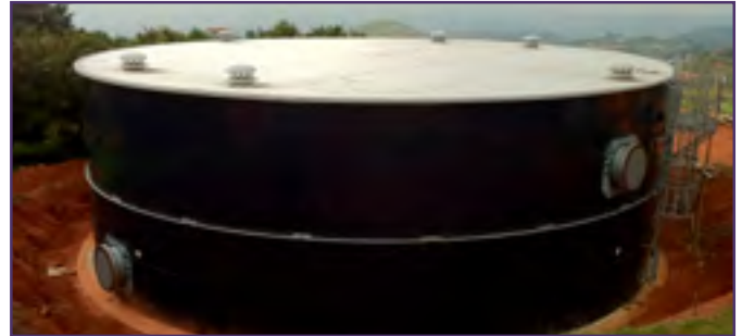
4: Trough Deck Roof – Drinking Water
