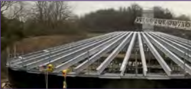
3: External Beam Roof – Anaerobic Digestion & Biogas
