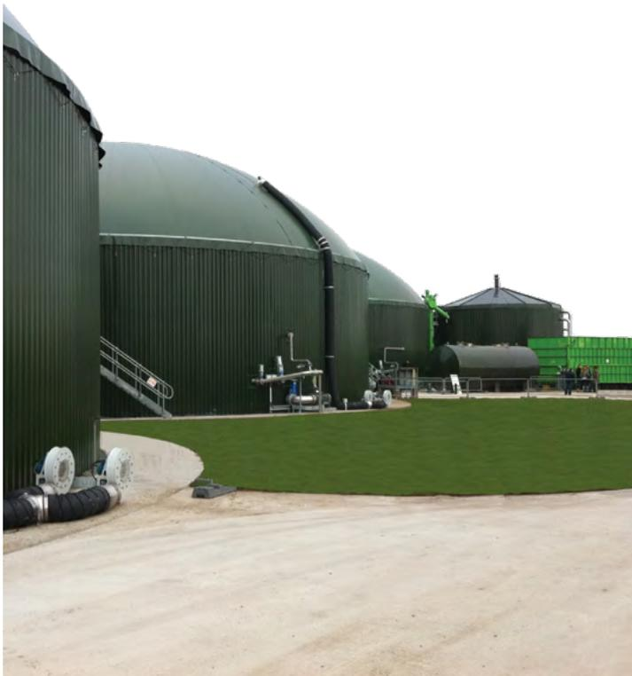
These roofs are structurally designed to allow for local environmental loading and can also support centrally mounted mixer systems.
