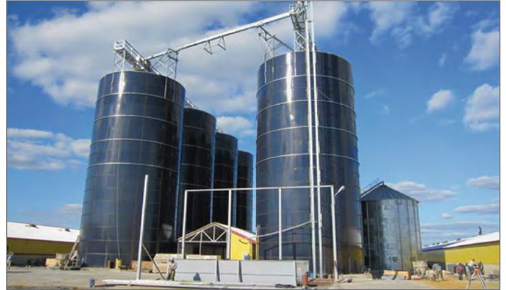
With a product history dating back to 1948, PERMASTORE® Glass-Fused-to-Steel silos provide clean and efficient storage of grains and forage. The secure sealed system of storage with capacities from 250 to 1400 metric tonnes (275 to 1540 US tons), gives significant benefits to livestock producers:
