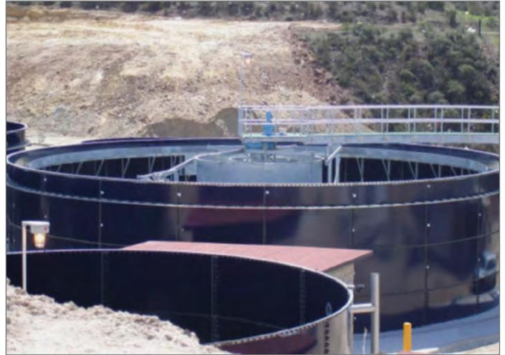
Glass-Fused-to-Steel tanks have a very high resistance to chemical corrosion and have excellent abrasion resistance properties, making them a suitable consideration in your sewage treatment application.
