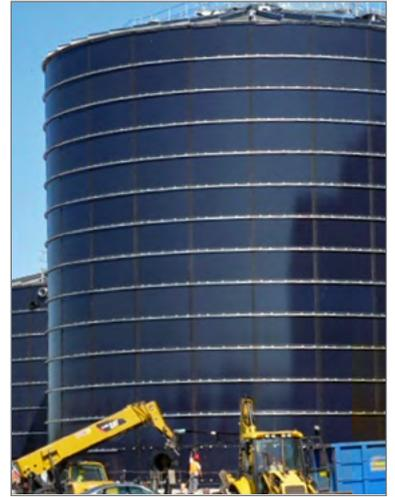
Tanks and silos are each supplied as a complete kit of components ready for assembly. The kit design includes features to ensure that the build can take place in the optimum time and be "right first time".
