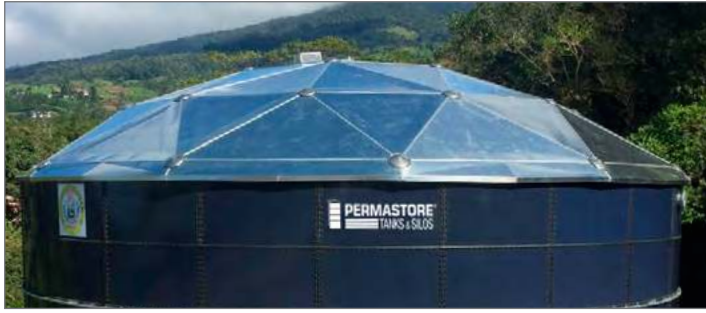
Geodesic Dome Roof – Costa Rica
