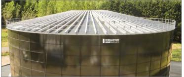
External I-Beam Roof – Anaerobic Digestion & Biogas
