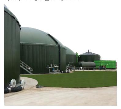
These roofs are structurally designed to allow for local environmental loading and can also support centrally mounted mixer systems.
